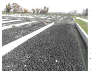
The sludge drying beds on site give an indication of the dimension of the FSM treatment problem, considering that the dried sludge can only be disposed of on the general waste dump side. The material represents an excellent bio-fertilizer or a good component for further co-composting with other organic matter. Unfortunately Jordanian regulations discourage the use of the product. Thus, charring the dried matter to produce biochar
