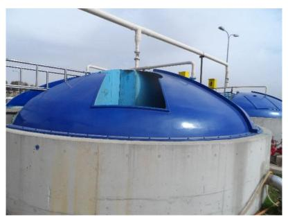
Ma'daba wastewater treatment facility: Several components were out of order and not brought back to operation, probably as they were not integral parts of the facility, particularly in terms of revenue generation. The picture shows two biogas out of order.
