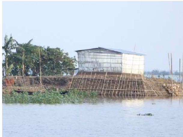
Protection with local stone and bamboo
