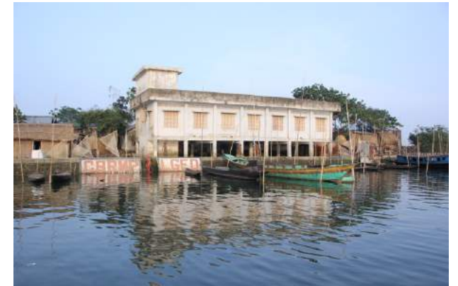
Protection with retaining wall
