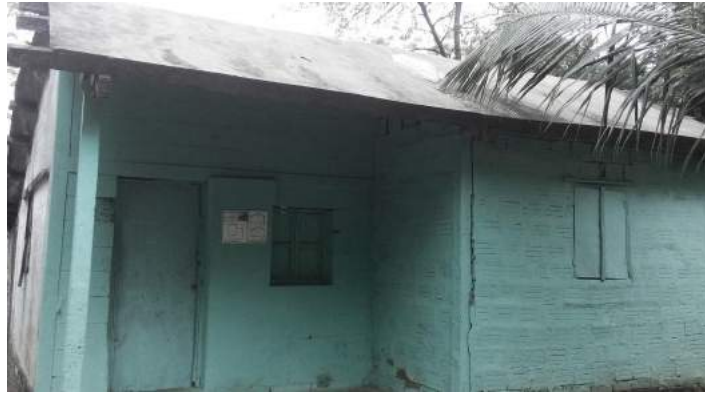
Cast in-situ Ferrocement Roof
