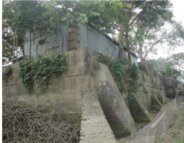
Protection with retaining walls along with buttresses
