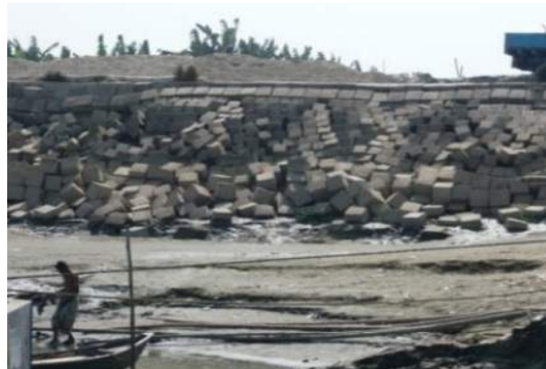
Concrete slope-stabilization blocks
