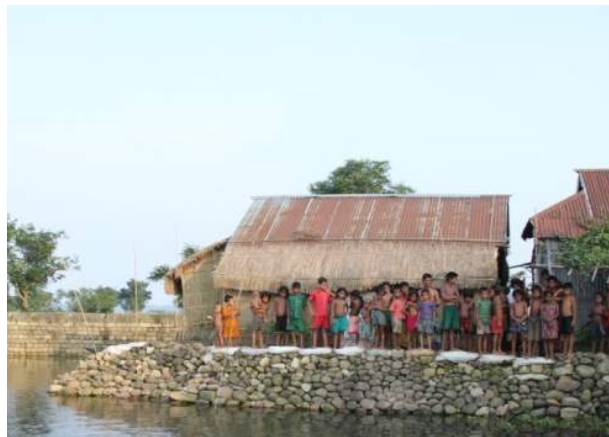
Protection with retaining walls and stones
