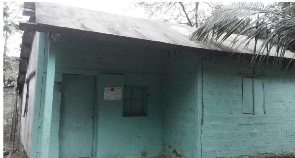
Cast in-situ Ferrocement Roof
