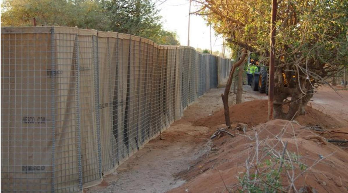
**Picture:** HESCO perimeter fence around DMO compound
