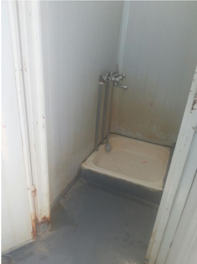
Figure 2: Shower block in WASH center, KAP refugee camp
