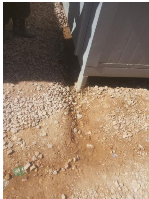
Figure 6: Trench dug to channel greywater exiting caravan
