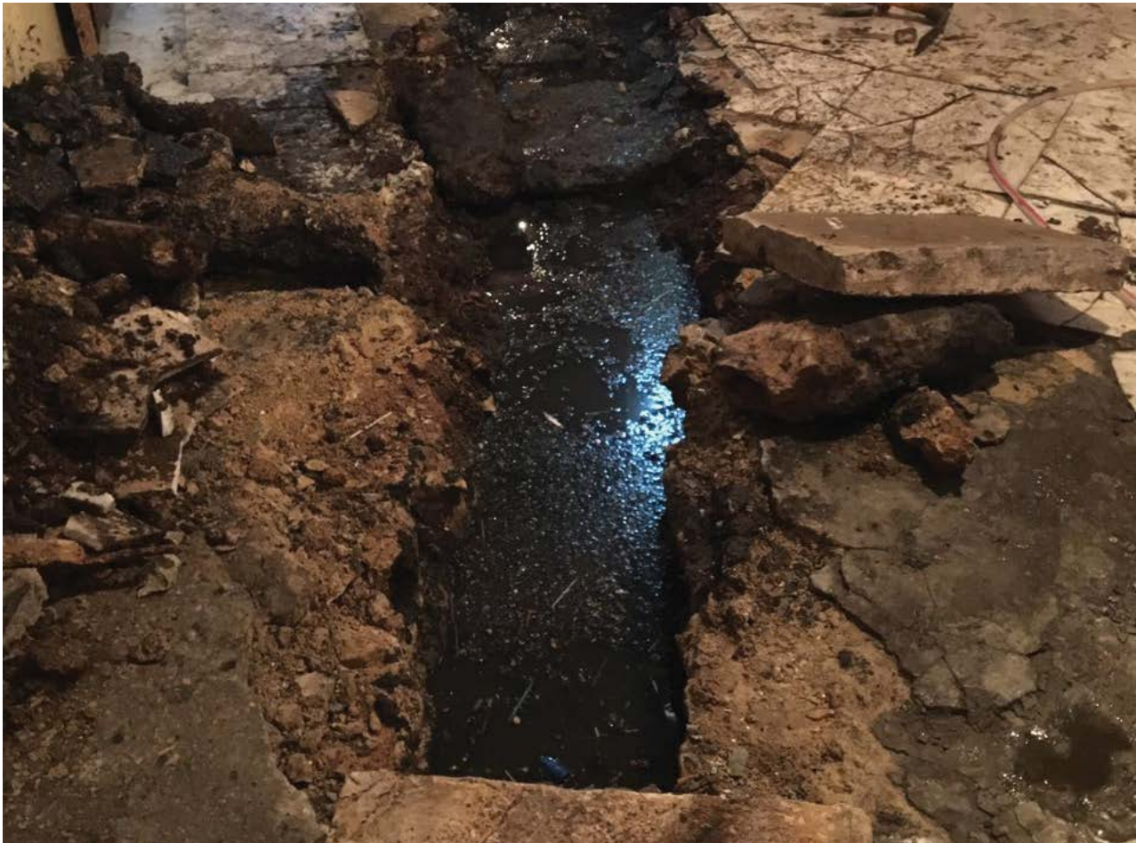
Ottoman sewer running under the tiles of what is now a dwelling house © Photo: Synne Bergby, UN-Habitat, 2016.
