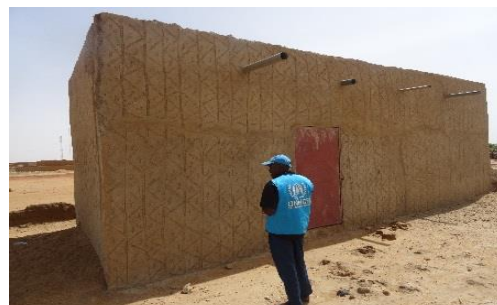
Mud shelter constructed for a returned refugee household from Niger in the region of Gao. © UNHCR
