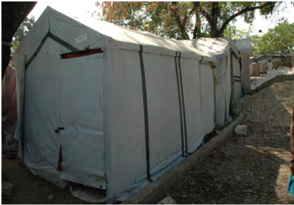
Site drainage improvements, protection for shelters at risk of water ingress along the slope.
