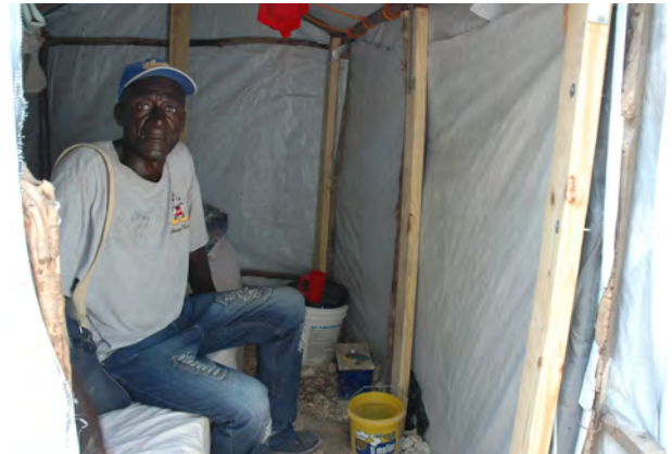
4 x 2 inch timber provided by CARE for shelter reinforcement, predominantly used to strengthen walls. Some families cut the timber to 2 x 2 inch sections.
