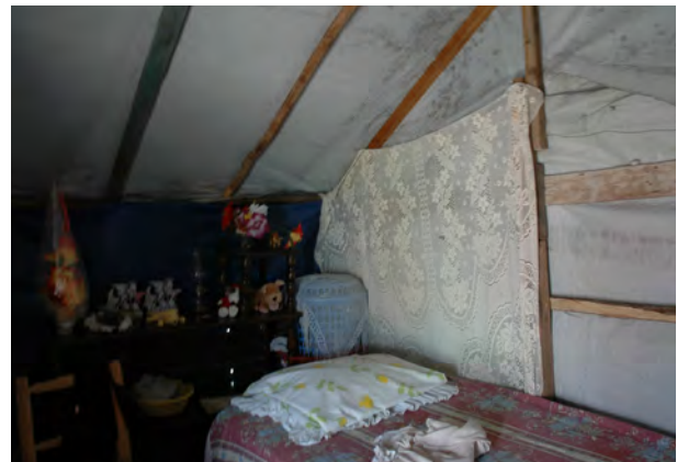
Roof and gable improved by technical support team, closer spacing of rafters.
