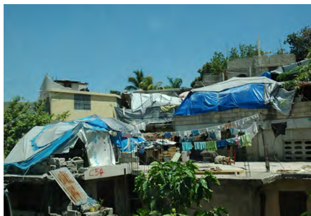
Two emergency shelters constructed on the roof of a damaged private house. Residents using the old house for storage and other activities, sleeping in shelter.
