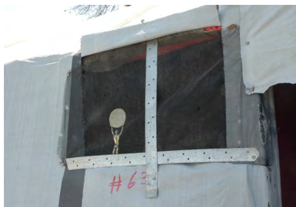
The same straps provided for hurricane reinforcement used to strengthen a window frame in a shelter. Residents used the straps in many ways.
