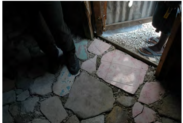
Doorway provides a threshold protecting the interior from site water. Internal floor leveled and raised with salvage materials.
