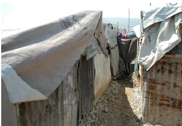
Good quality shelter grade plastic over self made shelter, used for roofing as waterproofing priority. Plastic damaged due to inadequate fixing.
