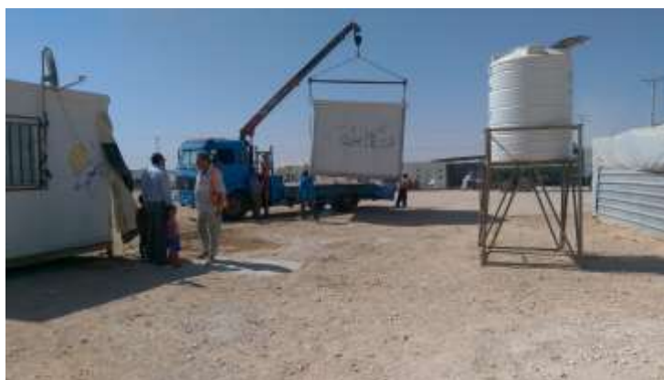
Fig. 2: Crane moving a caravan to ensure accessibility of the street.
