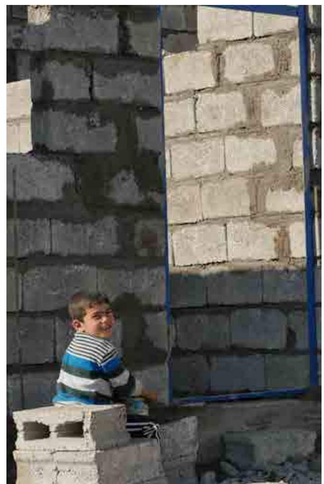
A refugee child is contemplating the construction of his new house in Gawilan Refugee Camp. Duhok, UNHCR/ R. Rasheed
