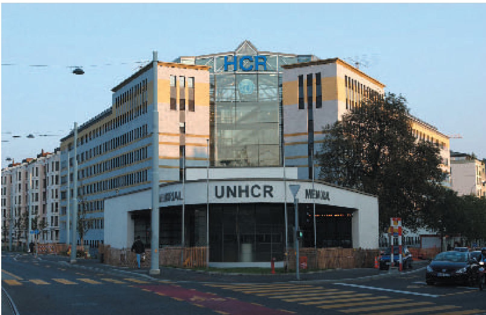
UNHCR Headquarters in Geneva, Switzerland. UNHCR / S. Hopper
