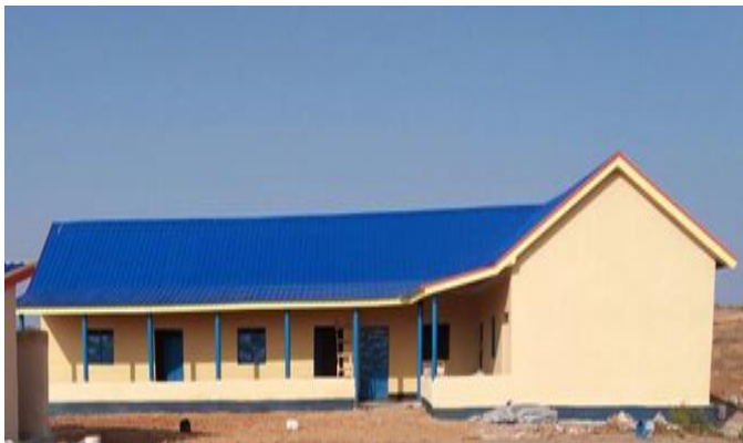
Construction of a Mother Child Health Centre in Kismayo as part of the integrated shelter project. © ARC/Kismayo, November 2017
