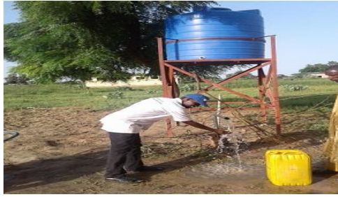
ACF converted borehole to solar
