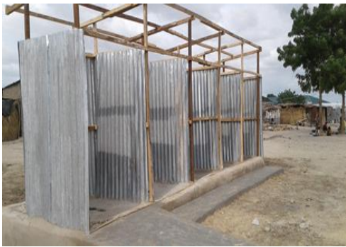
Construction of latrines by Fhi360 in the host community ongoing.
