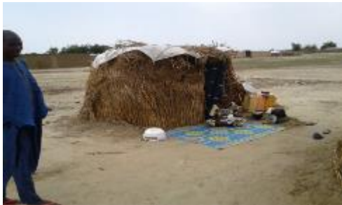
Makeshift needs renovation
