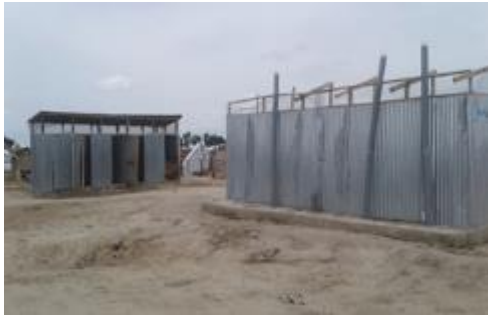
Abandoned Latrines on site
