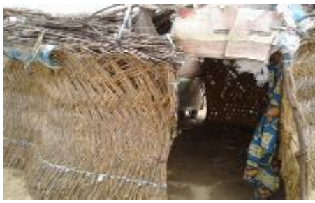
Makeshifts shelter that needs tarpaulins
