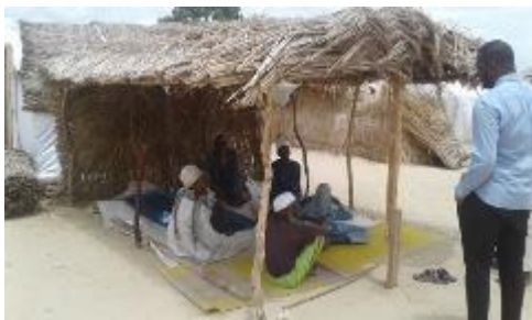
Mosque that needs urgent Tarpaulin Sheets
