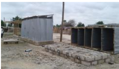
Renovation of latrine by SOLIDARITIES
