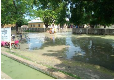
The only accessible hospital flooded with water
