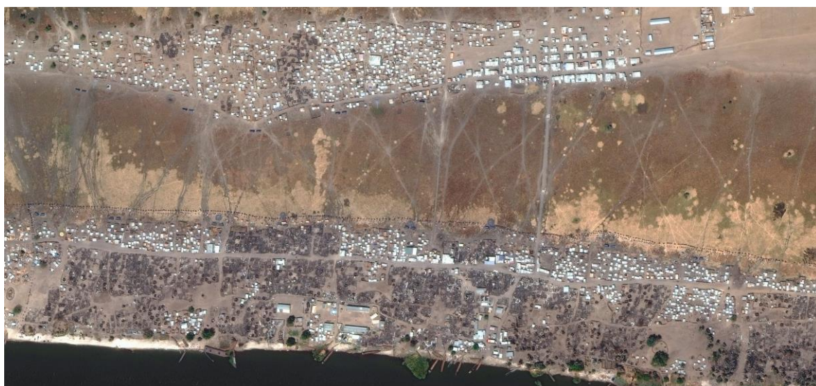
Imagery taken after 10 March 2017 shows burning and extensive damage of Wau Shilluk (at the bottom). The IDP camp has some damage as well. Coordinates: 9.661509, 31.742713, ©DigitalGlobe 2017, NextView License
