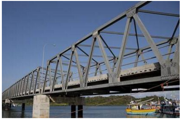
Trincomalee Bridge, China Bay
