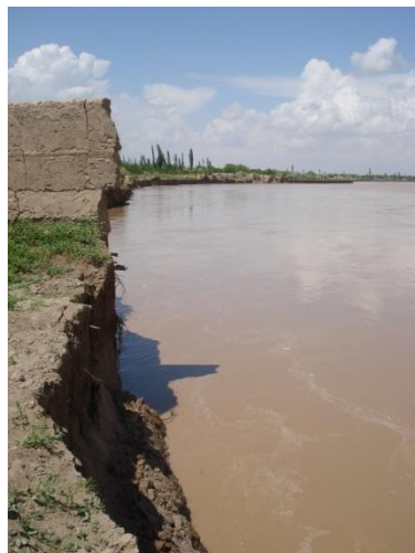
Amu river bank erosion Credit: OCHA Afghanistan
