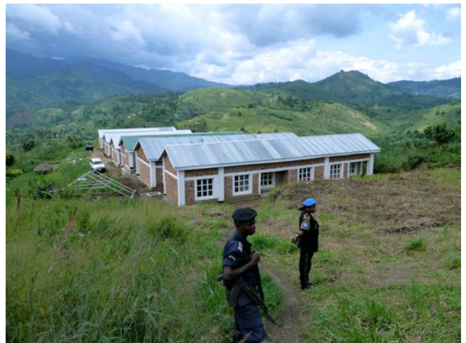
I4S police housing project in Bitale, South Kivu, 2014.
