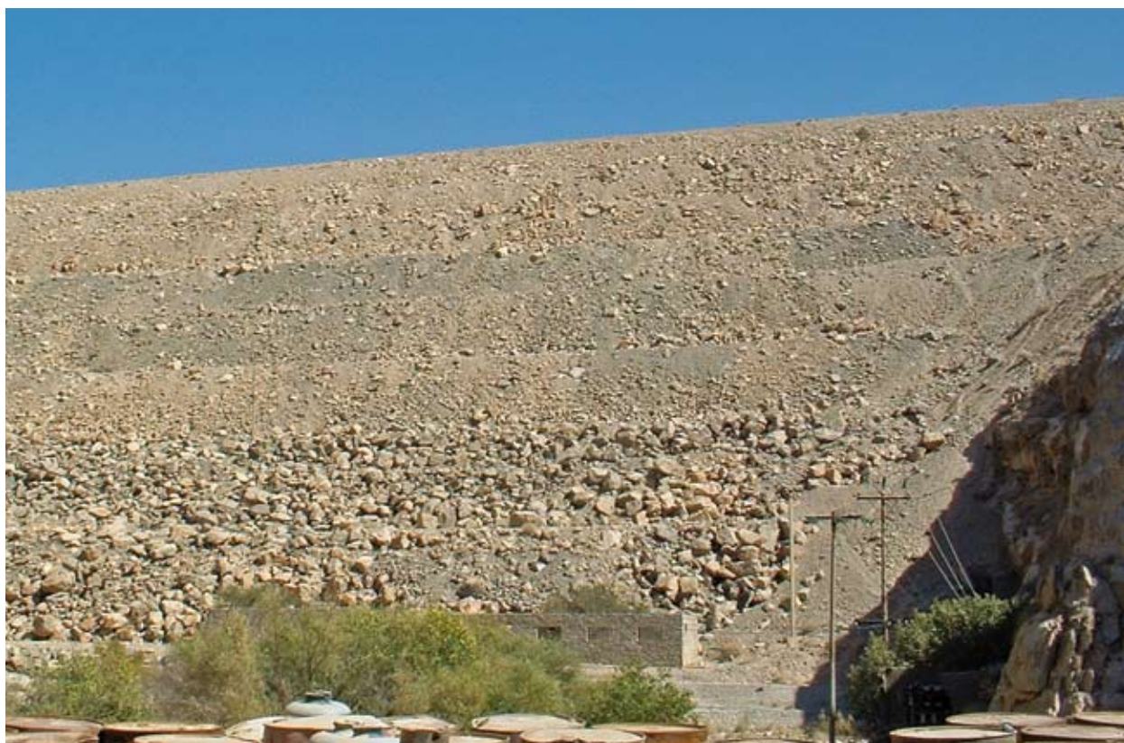
The reconstruction of the Kajakai Dam on the Helmand River has caused tensions with Iran
