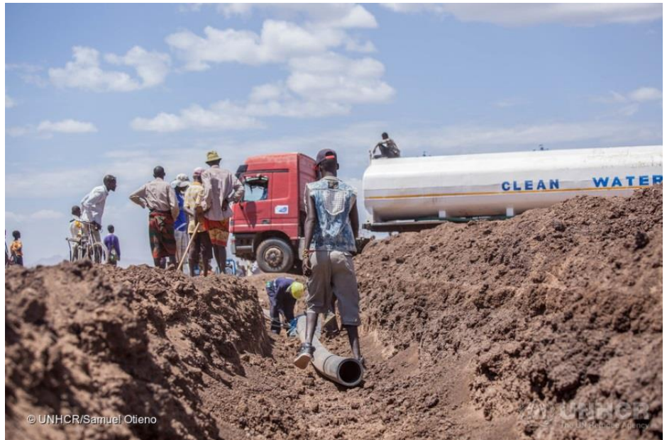
PHOTO: Ongoing laying and jointing of the 14Km water pipeline UNHCR/S.Otieno
