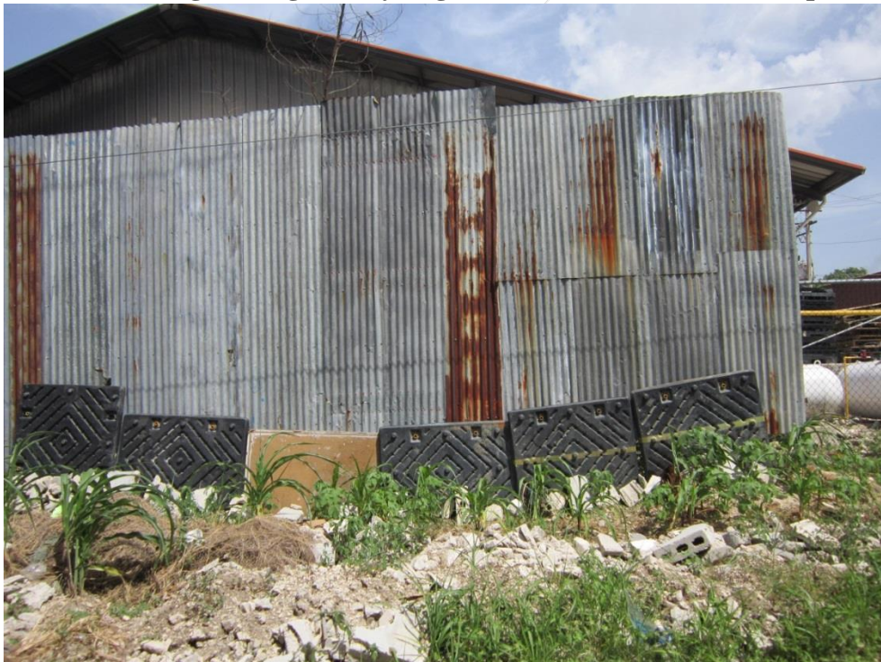
Figure 16.4 Detail of physical barrier created by case company to block heat, noise and fumes from neighboring factory in government-owned industrial park
