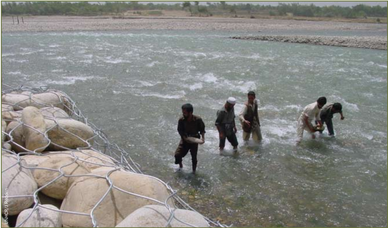
Returnee refugees building flood protection for Kalota, Kapisa Province, along Panjshir River, Afghanistan.
