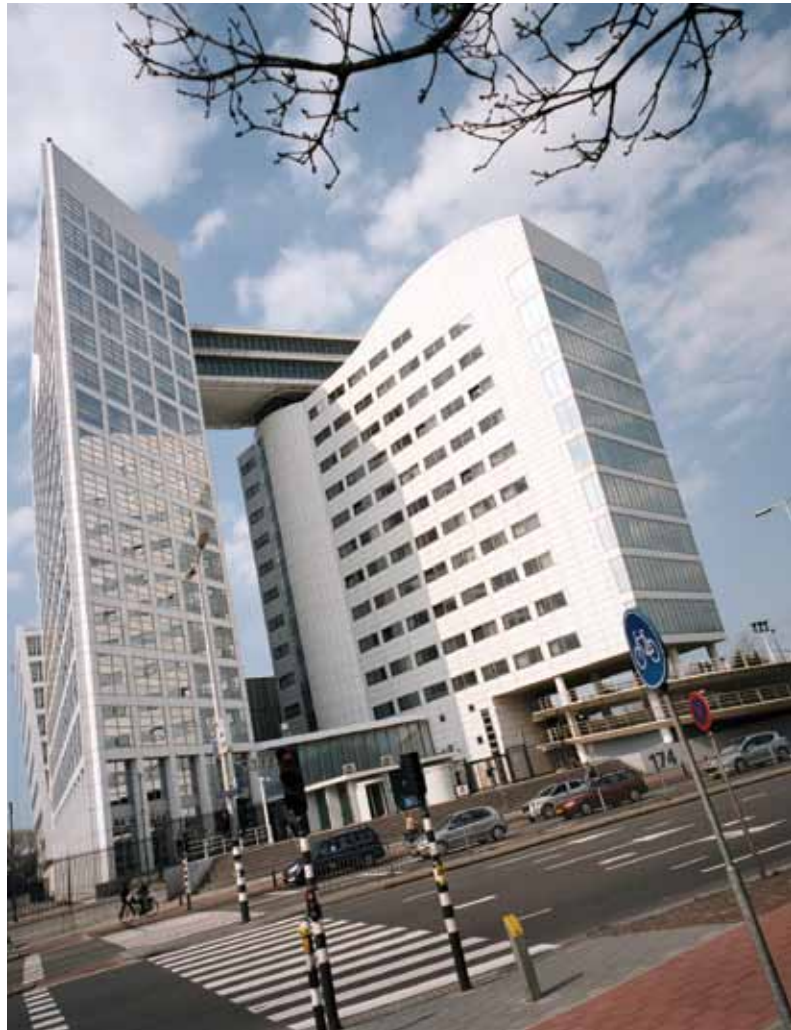
ICC Building. The Hague, Netherlands. © ICC-CPI/Max Koot
