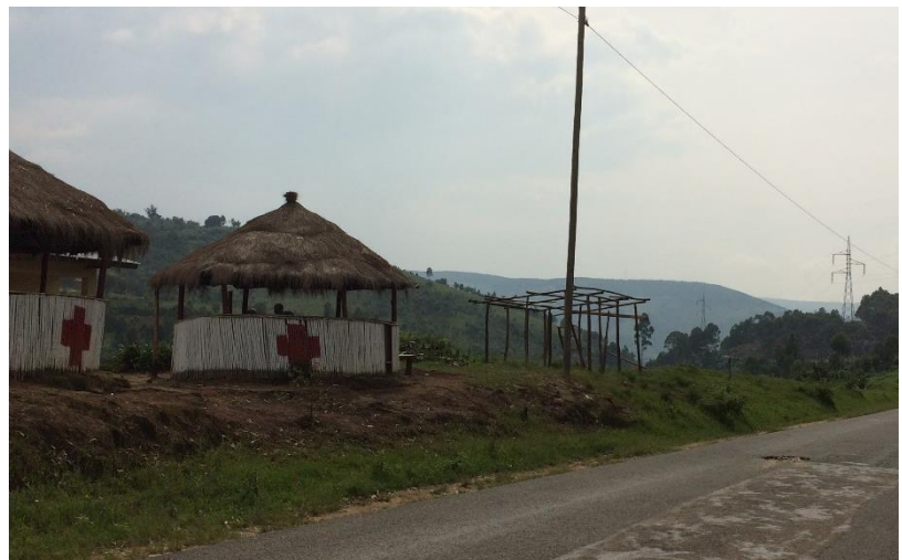
Road in Burundi, February 2016 © IRR/
