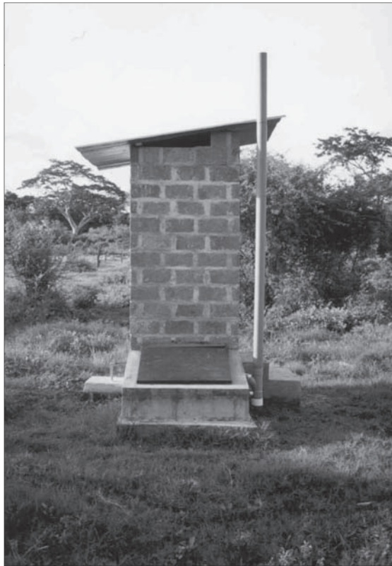
Photograph 5.1. Solar urine-diverting latrine in El Salvador
