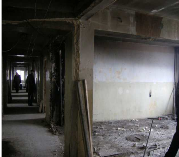
The renovation of reception facilities is underway
