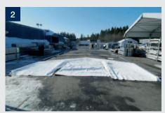
Install gable fabric on the ground before lifting to vertical position.\*
