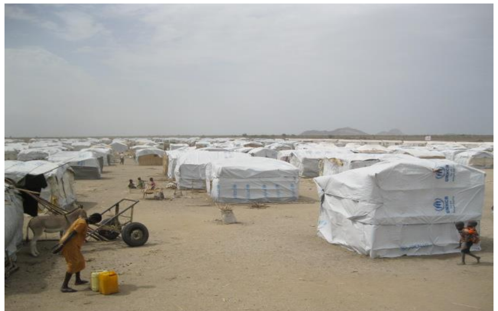
Improved shelter materials in Jouri relocation site, White Nile State. ©UNHCR / H. Abdalla / June 2014.
