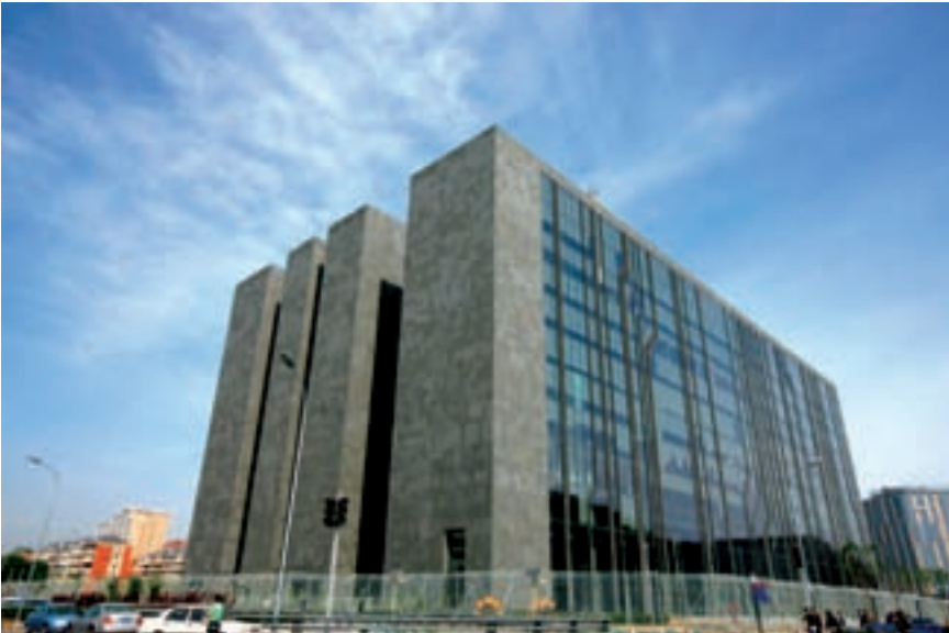
The Digital Beijing Building.
