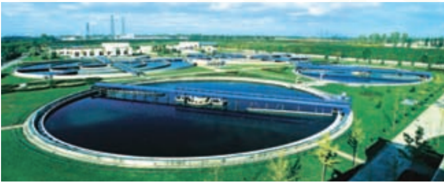
Gaobeidian sewage treatment plant.
