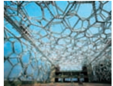
The steel structure of the National Swimming Centre (Water Cube).
