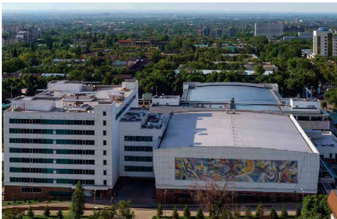
Baluan Sholak Sports Palace, Central Cluster, ice hockey 2, existing
