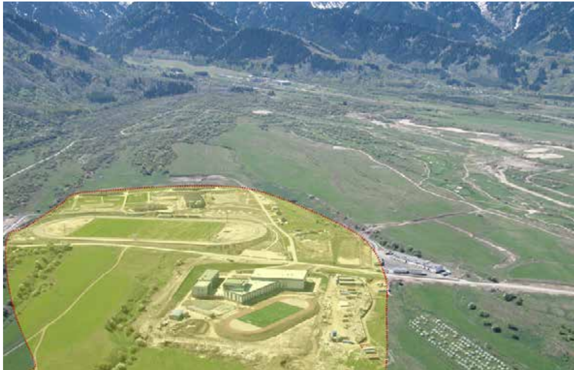
Ak Bulak, Al Bulak Cluster, Olympic Village, to be built
