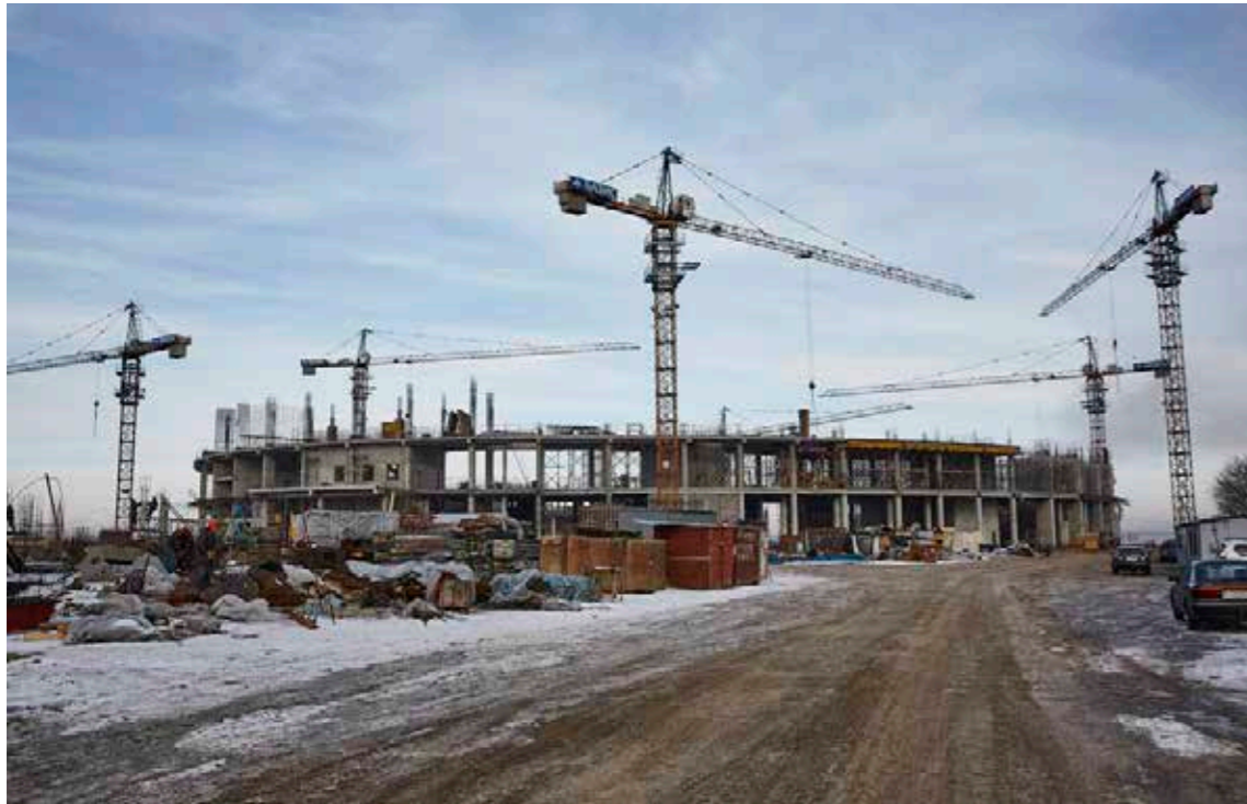
Ice Palace, stand-alone venue, ice hockey 1, under construction
