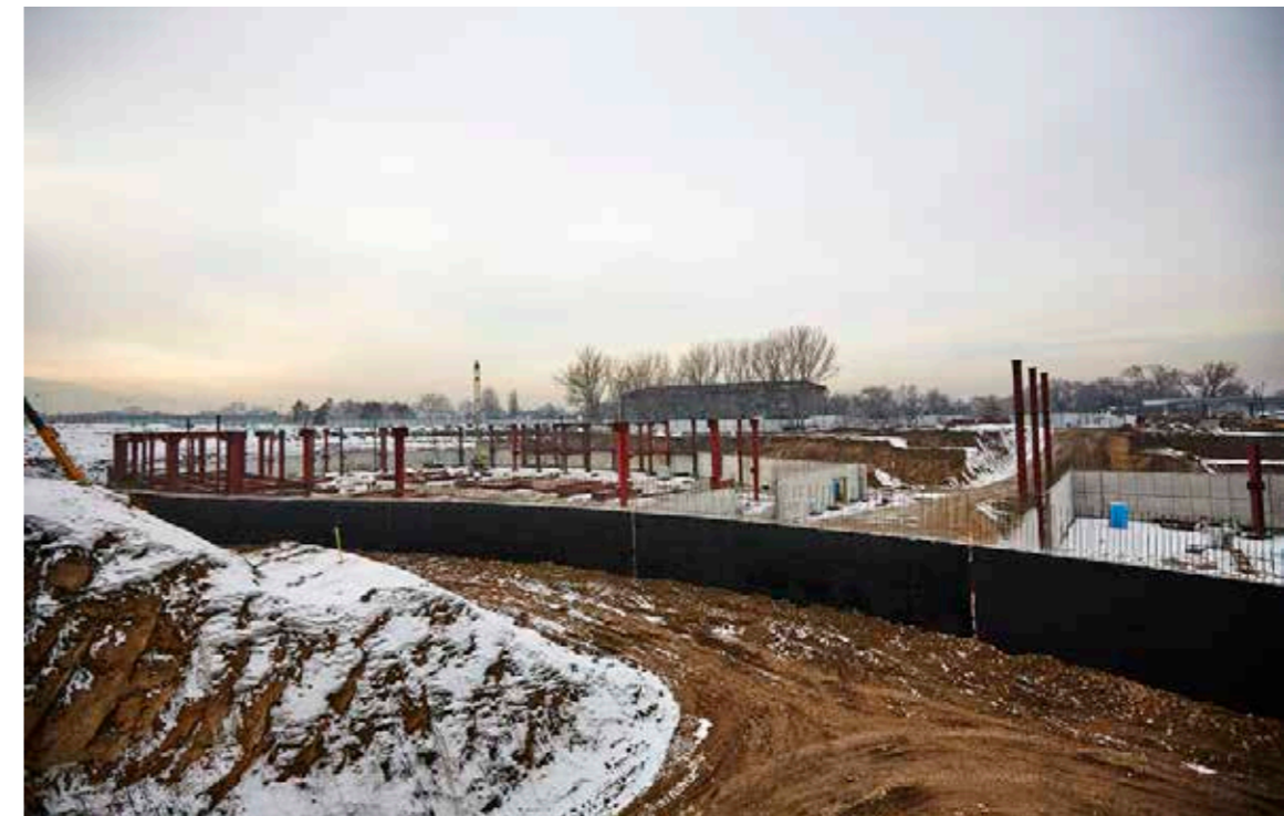
Curling Arena, stand-alone venue, curling, under construction
