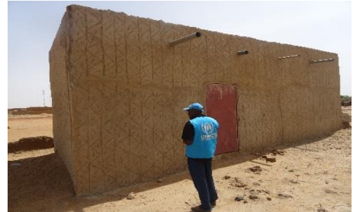
Mud shelter constructed for a returned refugee household from Niger in the region of Gao. © UNHCR
