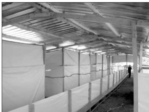
Site design should foster the logical flow of people through the registration process.
