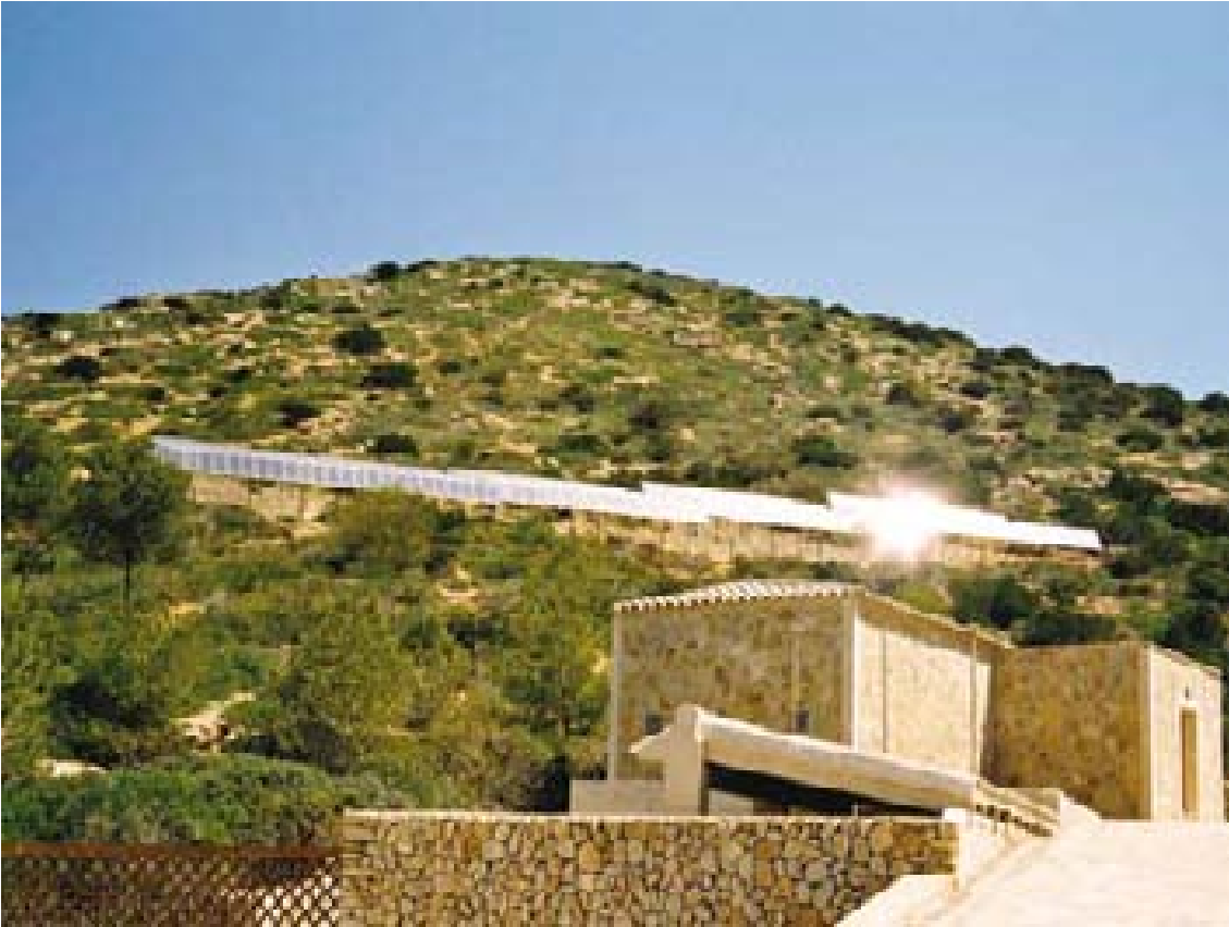
Figure 26: In countries with high sunshine levels, solar panels are particularly suitable for providing electricity for sports or other isolated facilities (Island of Cabrera, Balearics, Spain).
