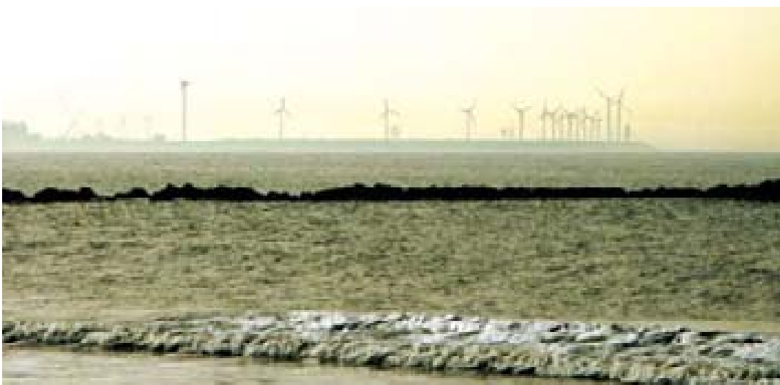
Figure 15: Wind turbines at the entrance to the port of Ostend (Belgium).
