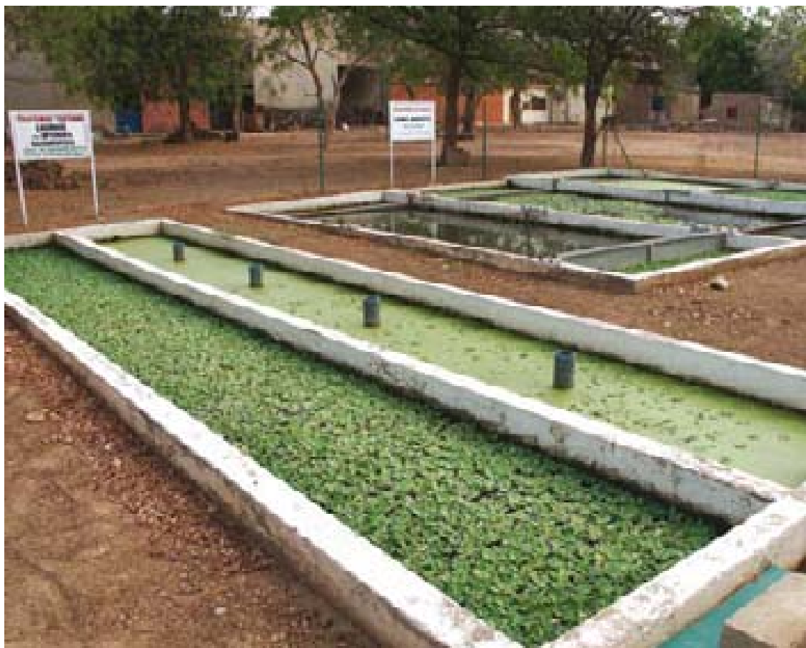
Figure 6: Treatment of waste water in Africa (Burkina Faso) by phytopurification.
