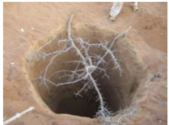
A refugee-dug pit ready for slab
