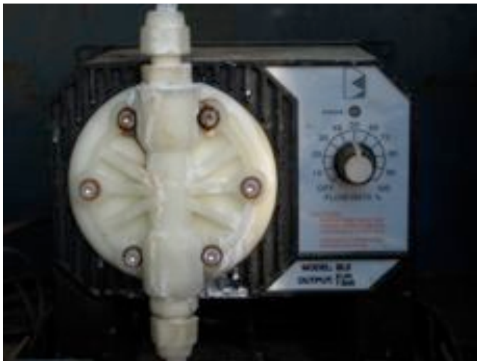
An automatic chlorinator and the 1% chlorine solution that feeds the chlorinator
