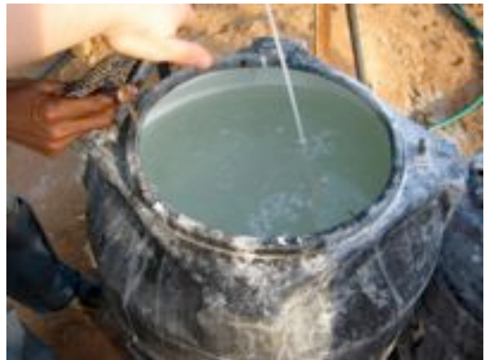
An automatic chlorinator and the 1% chlorine solution that feeds the chlorinator
