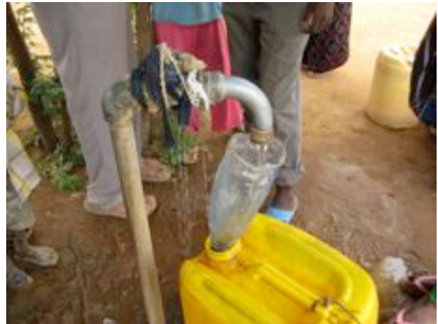
A (working) flow meter and a very leaky tap
