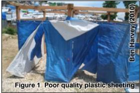
The use of plastic sheeting toilet superstructures is an emergency solution and must be phased out after the first six months of any response. Flaps of plastic sheeting may be used in the initial first phase response provided they are adequately weighted at the bottom of the flap and they are phased out within 3 months. Female blocks with plastic flap doors should be equipped with a privacy screen.
