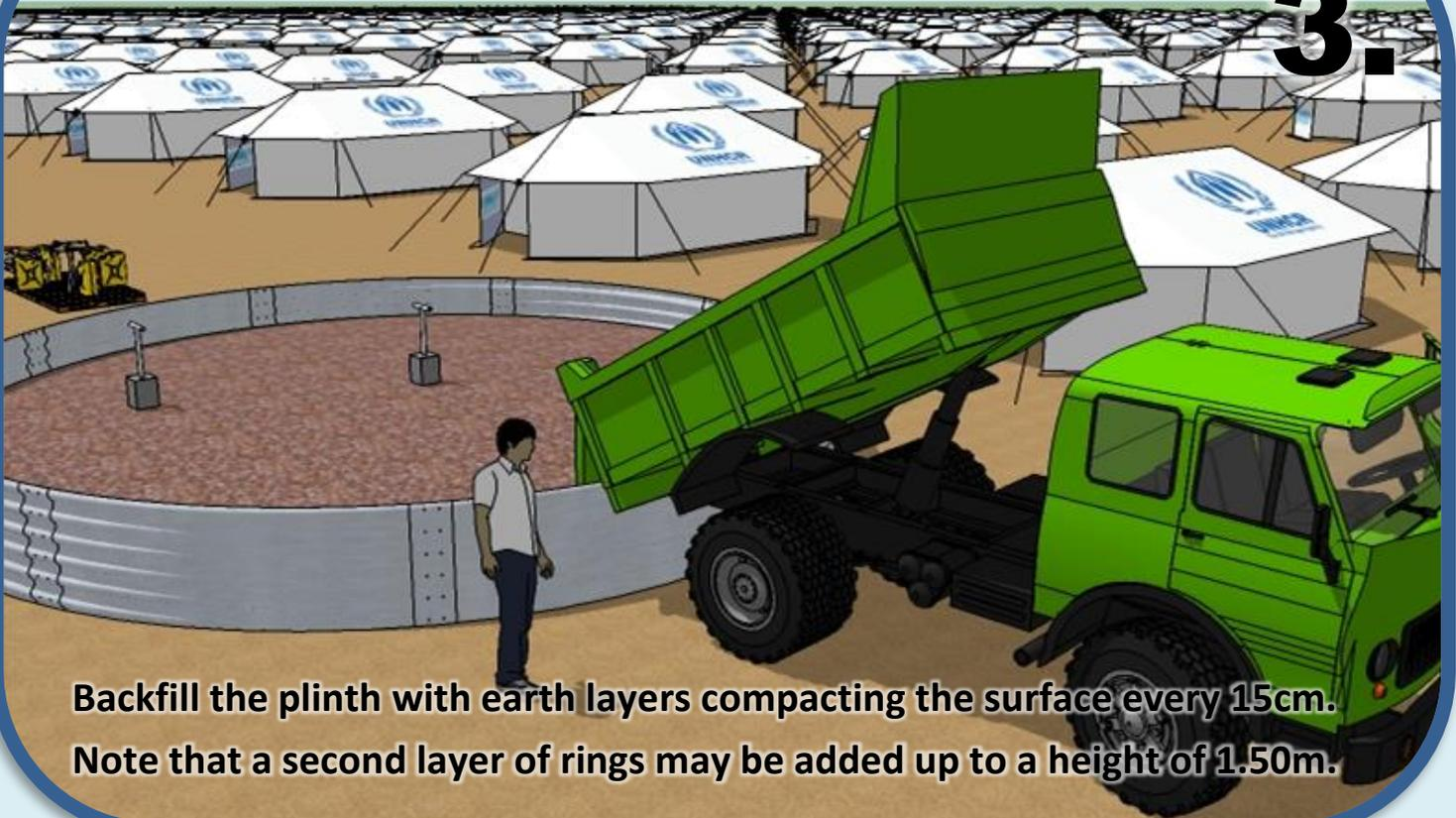
**Backfill the plinth with earth layers compacting the surface every 15cm. Note that a second layer of rings may be added up to a height of 1.50m.**
