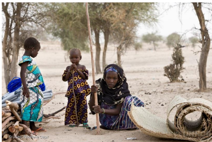
Niger/Nigerian refugee Boussam, 15, installs a pole to start building her new shelter in Sayam Forage Camp, Diffa Region, Niger © Hélène Caux/ 11 May 2016
