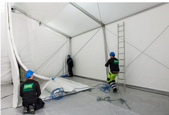
Follow the same procedure to lift the cover to the corner. Pull the ropes and hold until its fixed.
