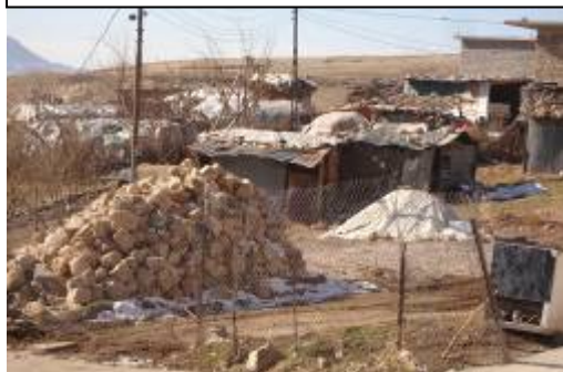
Two-room IDP shelter with makeshift roof in Sumel District, home to a family of four. Rent: US $200 per month.
