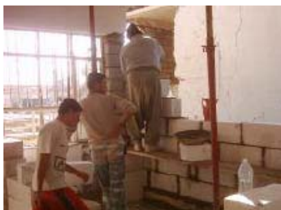
UNHCR shelter rehabilitation Programme in Mosul (2008)
