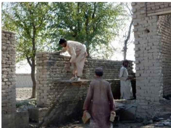
Figure 2: Refugees constructing shelters in Village B Mandozai
