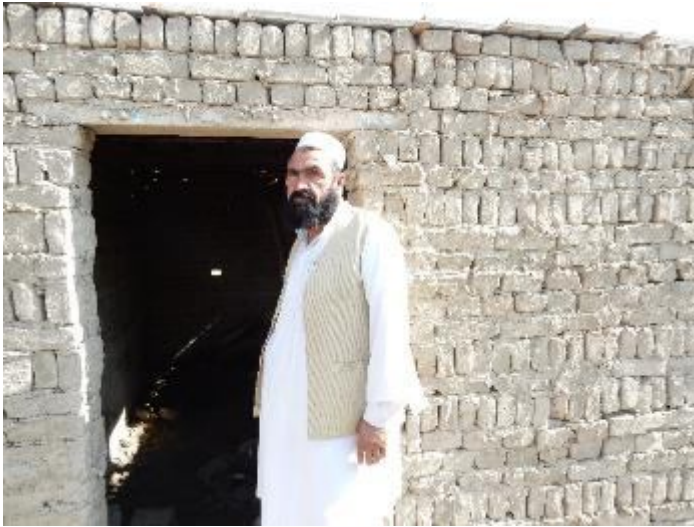
Figure 3: Sahir in front of a transitional shelter under construction
