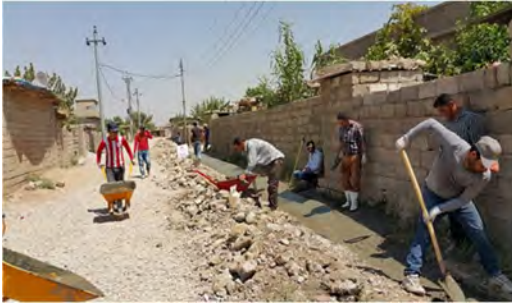
Construction of open channels in Husseiniya Settlement (UNHCR/H. Fahmi)
