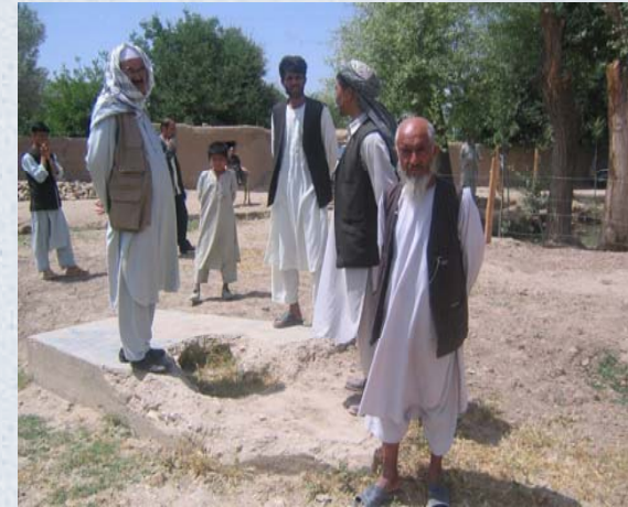
WP reported as damaged
