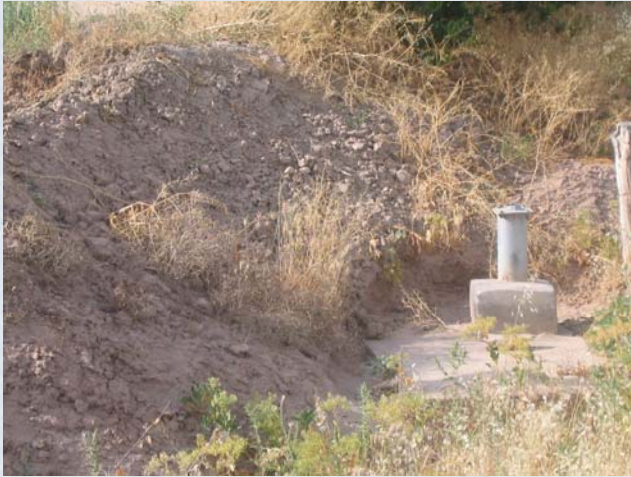
WP left abandoned due to less water
