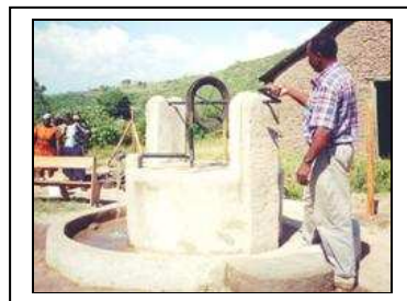
Protected hand dug well with hand pump
